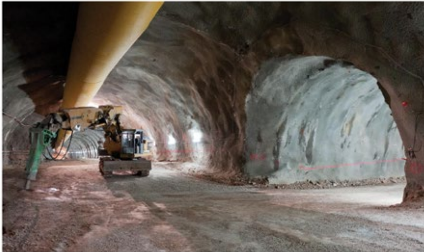
Autoroute Corinthe-Patras Tunnels Panagopoula
